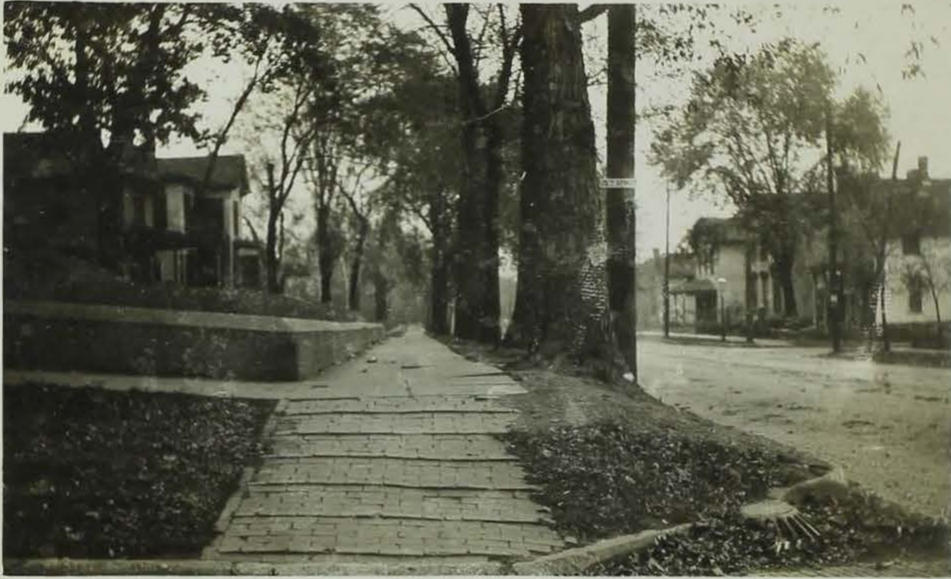
15" Woodland An illustration of old-fashioned sidewalk, catch basin, and corner curb in a high class residence section of Des Moines.
