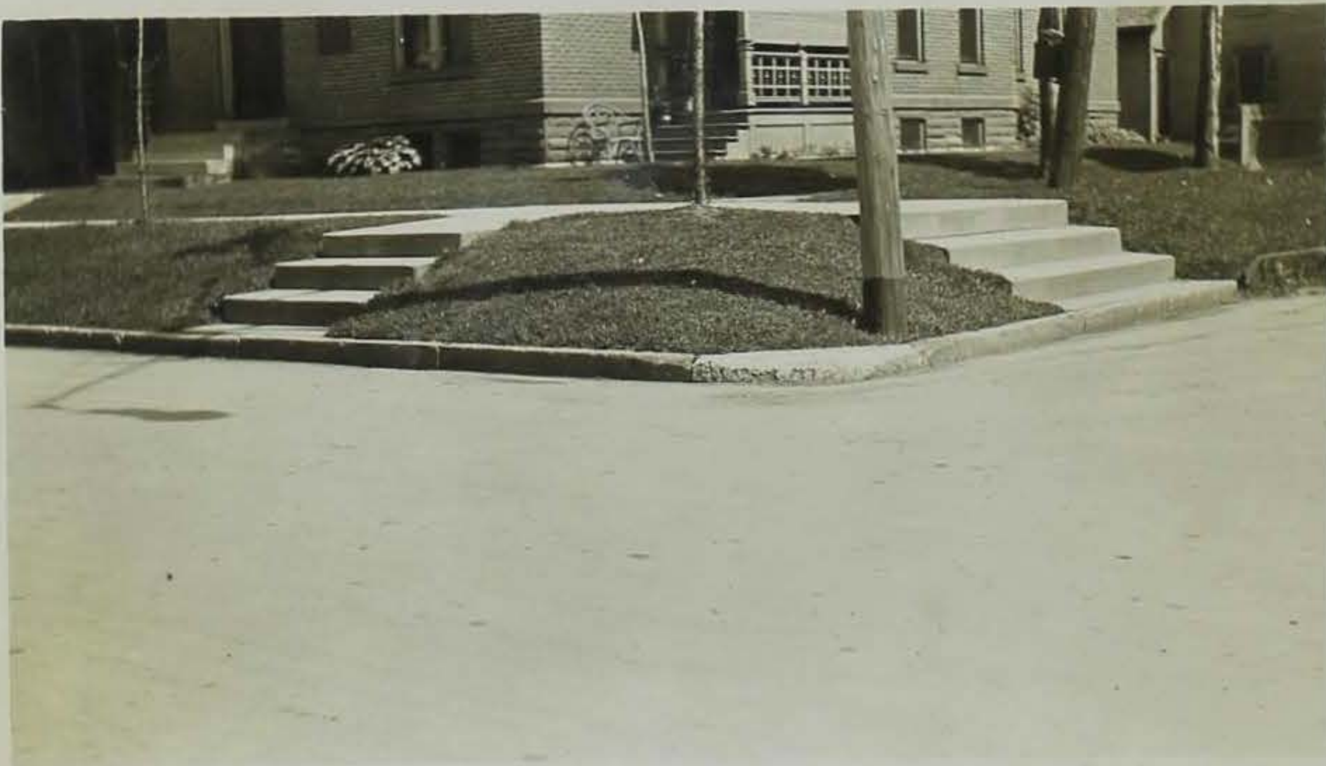
Better handling of a like problem, though here the radius of the curb at the corner is too small. Photograph from Fort Wayne.
