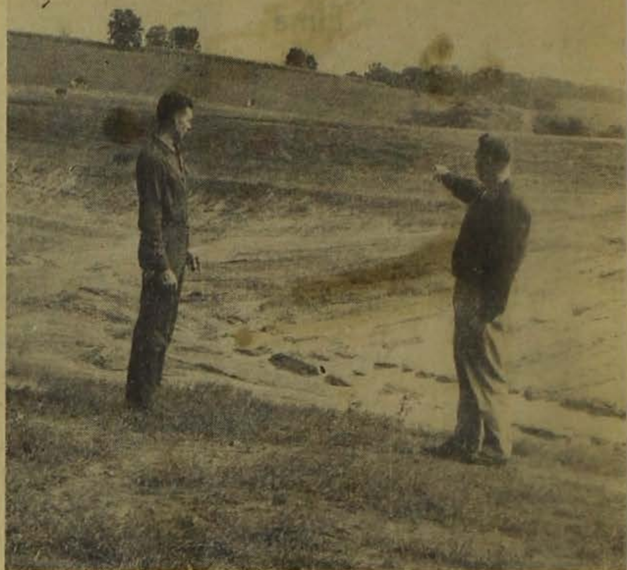
GENE FARMER (left) and Cal Moore, both of Eldora, look over the large earthen-fill erosion control structure which will fit into the conservation program for the Pine Lake watershed. The "drop inlet" structure is on land owned by the
