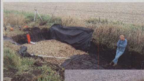
An Underground Outlet during construction . .
