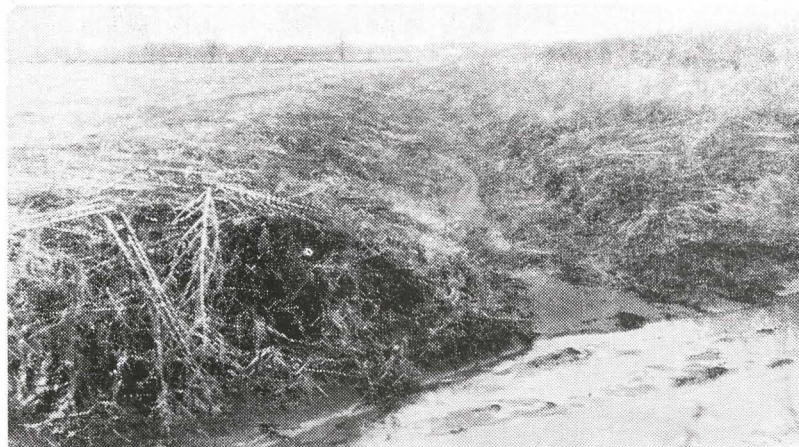
This drainage ditch in the Moulton Watershed was put in cooperatively by Mrs. Lettie Daniels and Doyle Anderson to provide an outlet for drainage of the bottomland shown.
