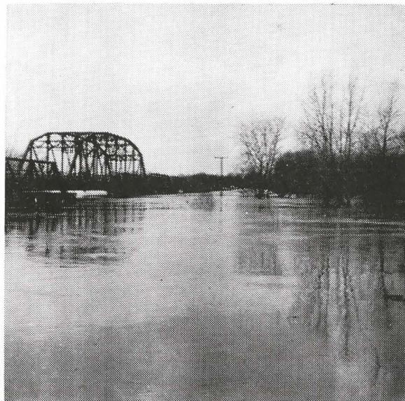
Highway No. 2 river bridge, a familiar scene. The Chariton River in full spring flood. Through the development of watersheds in the upper tributaries, much of this flooding can and will be controlled.
