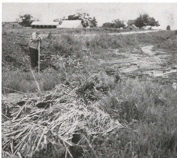
Upstream side of county road culvert near Charles McDanolds' farm, Little Walnut Watershed, showing roadside erosion and siltation deposits.
