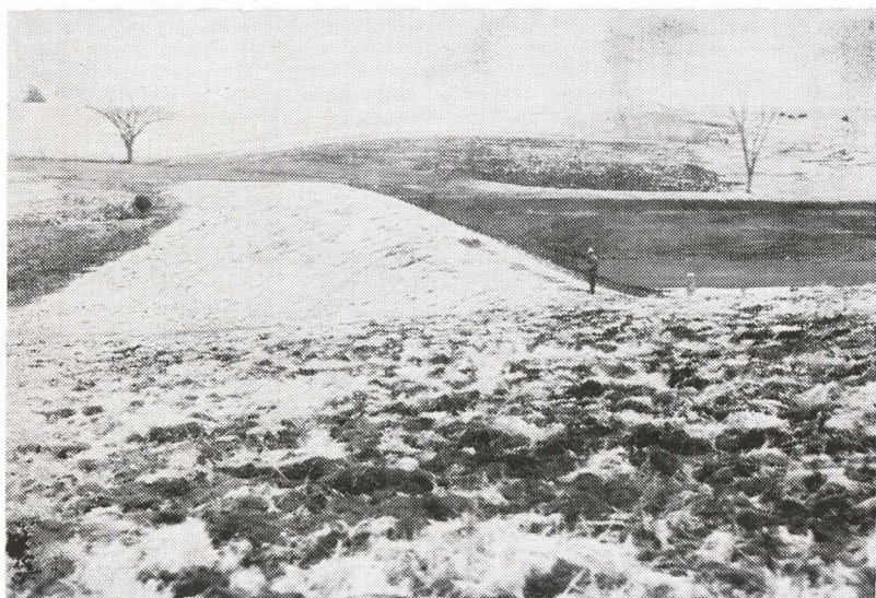
This picture taken at the Cliff Singley farm, Fox Watershed, shows old pasture in the foreground which has been brush disced preparatory to renovation. The structure in the background was constructed in an old gully to halt the progress of erosion. As can be seen in the picture, the structure fill has been very thoroughly mulched for protection until the seed has a chance to take over.
