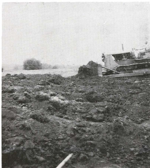
Graded terrace construction on the Dallas Walker farm, Walnut City Watershed. This picture shows the first pass of the bulldozer pushing up the initial ridge.
