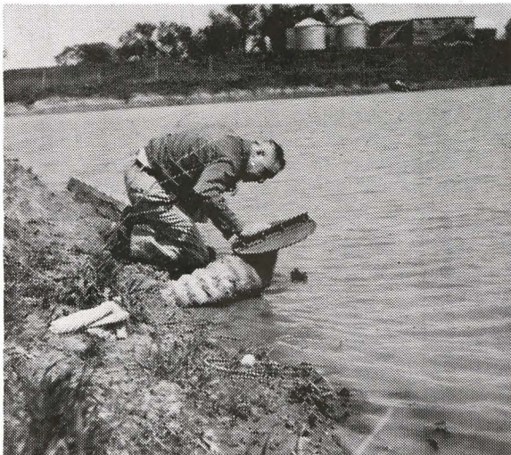
Hood-inlet in the Charles McDanolds' farm directly below the road culvert. This eight-inch hood with two-foot impoundment stage contained all the water which twice washed out the county road culvert in the spring of 1960.
