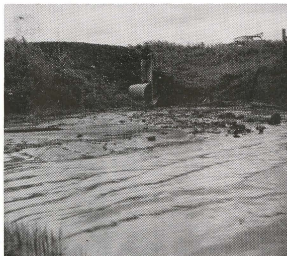
Downstream side of same culvert showing a thirty-six-inch culvert and deposition of silt in the pond area.
