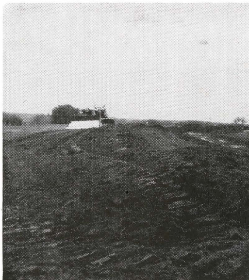
Contractors' first finishing step down the channel of the terrace on the Walker farm. This step in the finishing process will leave the terrace with a ten-foot channel.
