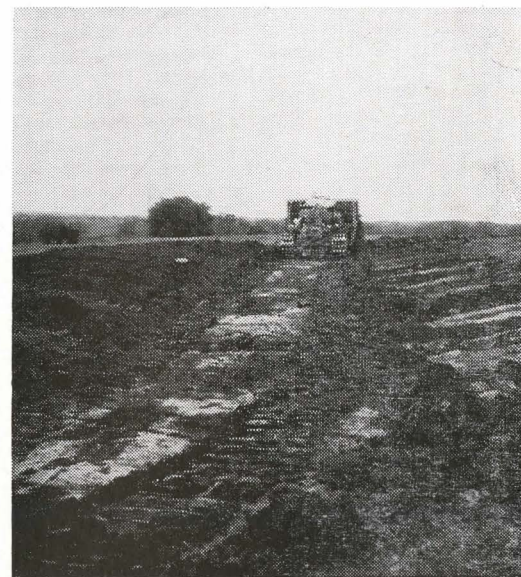
The final finishing pass on the Walker terrace. In the picture the contractor is smoothing the back slope and at completion the terrace is ready to be farmed with the rest of the field.
