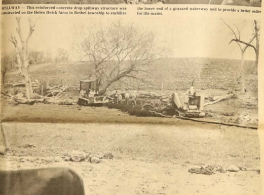
SPILLWAY — This reinforced concrete drop spillway structure was constructed on the Helen Hick farm in Bethel township to stabilize the lower end of a grassed waterway and to provide a better outlet for tile drains.
