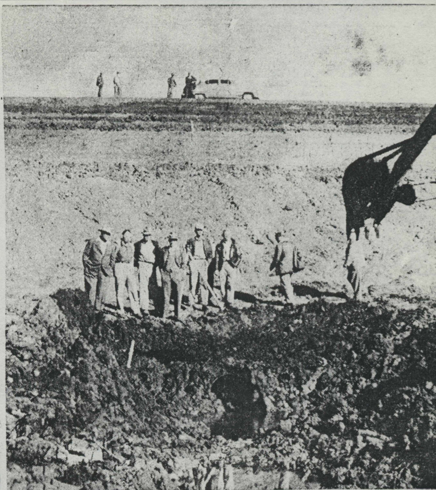
The Outlet . . . of the overflow tube on the downstream side of control structure County Farm is inspected by county supervisors and SCS engineers.—Nonpareil PH
