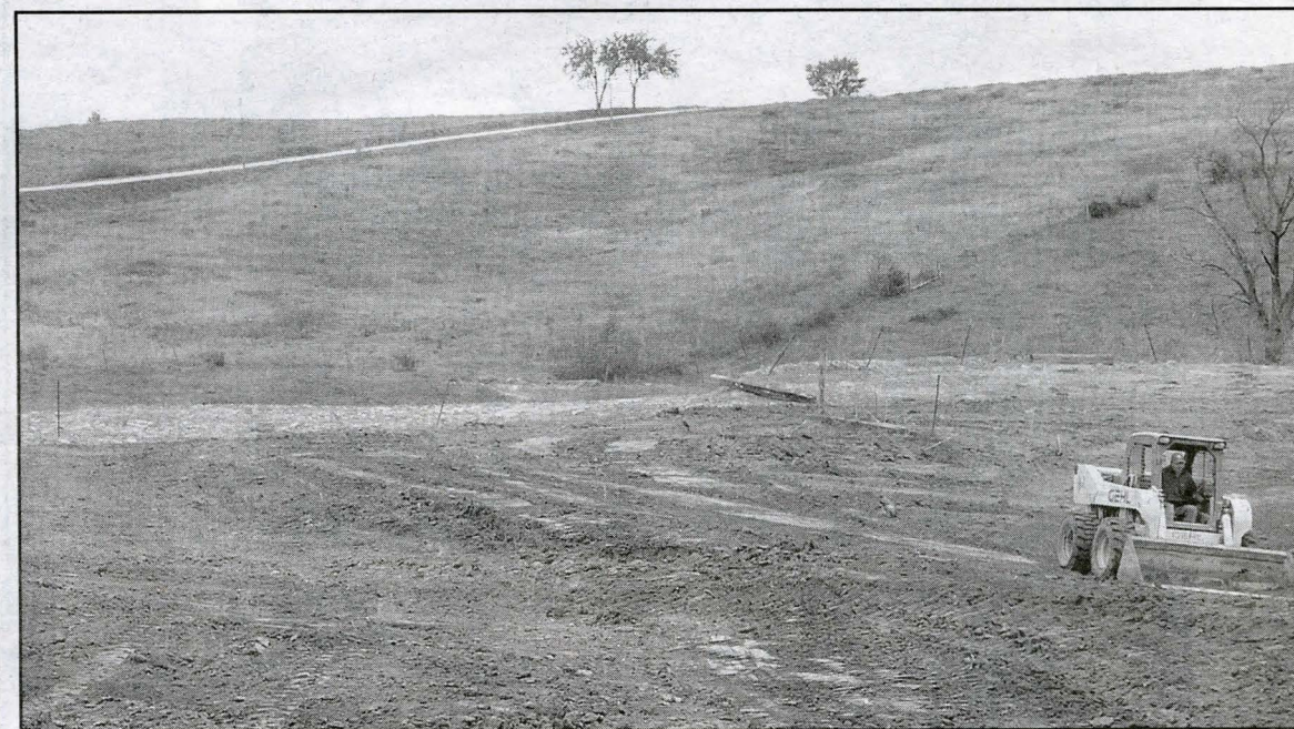
A grassed filter strip constructed at Mike Baumler's during construction of the cattle lot. This grass filter strip filters runoff from the settling basin water and the milk house water runoff.
