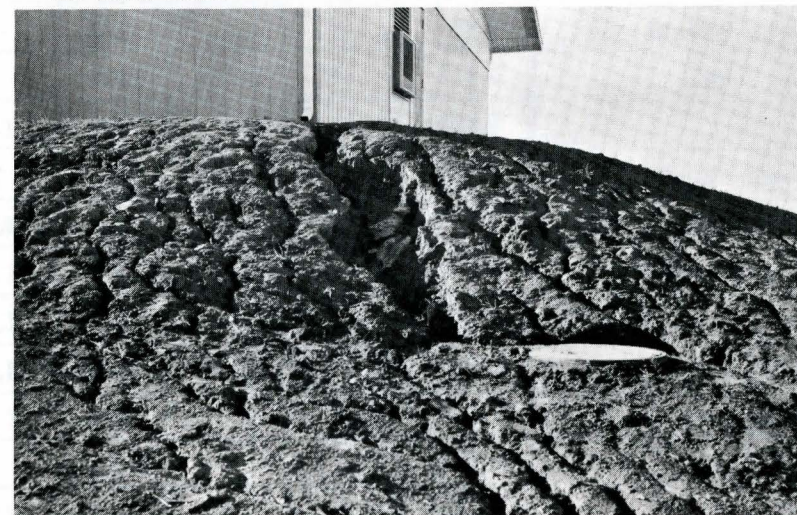
Soil erosion endangers an "instant campus" building at the Indian Hills Community College at Centerville, Iowa. Critical areas such as this sparked a college request for erosion control assistance through the Chariton Valley Resource Conservation and Development Project. RC&D County Steering Committee members and their field of representation are: Bill Dillon, Centerville, Chairman, Business; Leon Kauzlarich, Mystic, Soil Conservation District; Doyle Anderson, Moulton, County Board of Supervisors; Lee Benz, Moravia, Agriculture; Henry Little, Centerville, Civic Groups; and Boyd O'Briant, Centerville, Industry.
