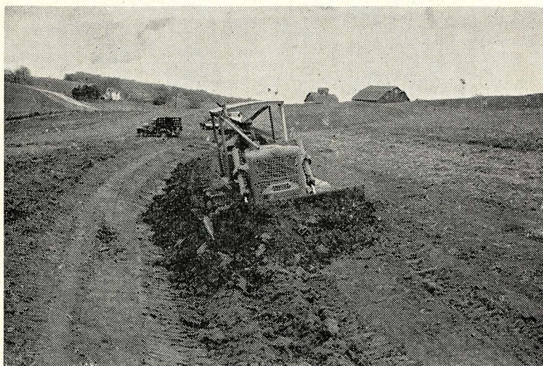
Building a terrace with bulldozer, Earl Eiselstein farm, Massillon Township. Terracing gives the best erosion control of the mechanical practices.
