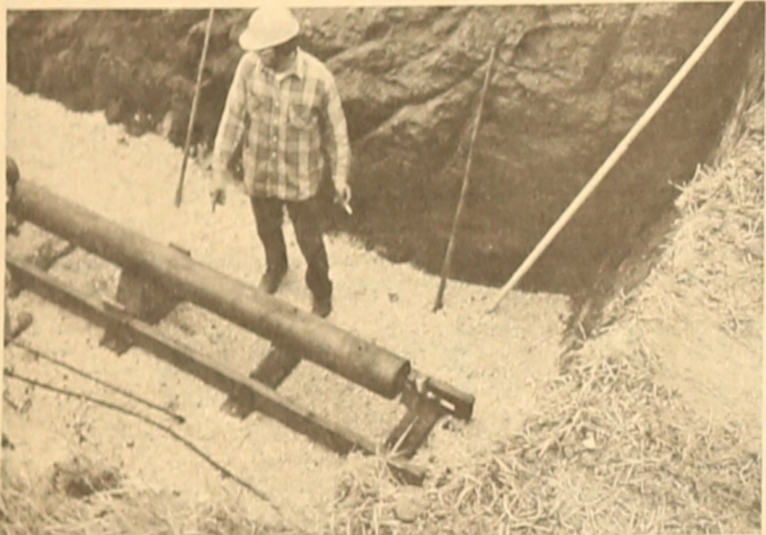
AUGERING — The next step is augering under the hard portion of the road. The auger moves on a track which must be graded to give the pipe the proper angle so that when it reaches the opposite side it will have sufficient grade and depth.
