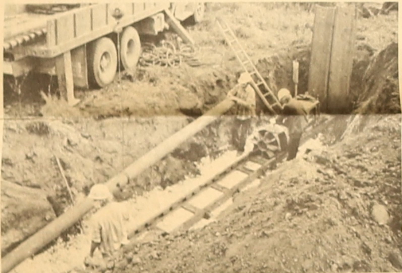
SECTIONS — As augering proceeds, sections are added. After the hole has been made, corrugated metal pipe sections are then pushed in place. Cost of this work was paid by the Iowa State Highway Commission.
