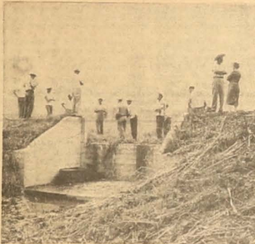
CONSERVATIONISTS and interested farmers observe a drop spillway, tile outlet on the Art Malt farm in Clermont township. The spillway is used to stop a gully and is located at the bottom of a grass runway. Malt also takes advantage of the tile outlet for livestock watering.
