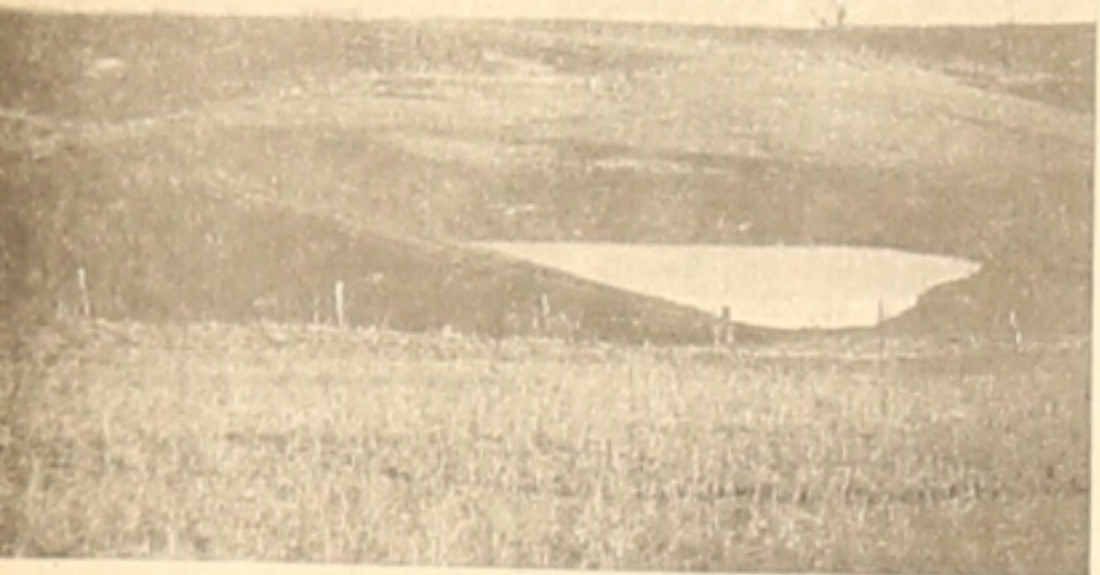
PICTURED IS THE RECENTLY COMPLETED erosion control structure on the Richard Meyer farm in Dover township. The dam was used to control a gully and stabilize an eroding roadway.
