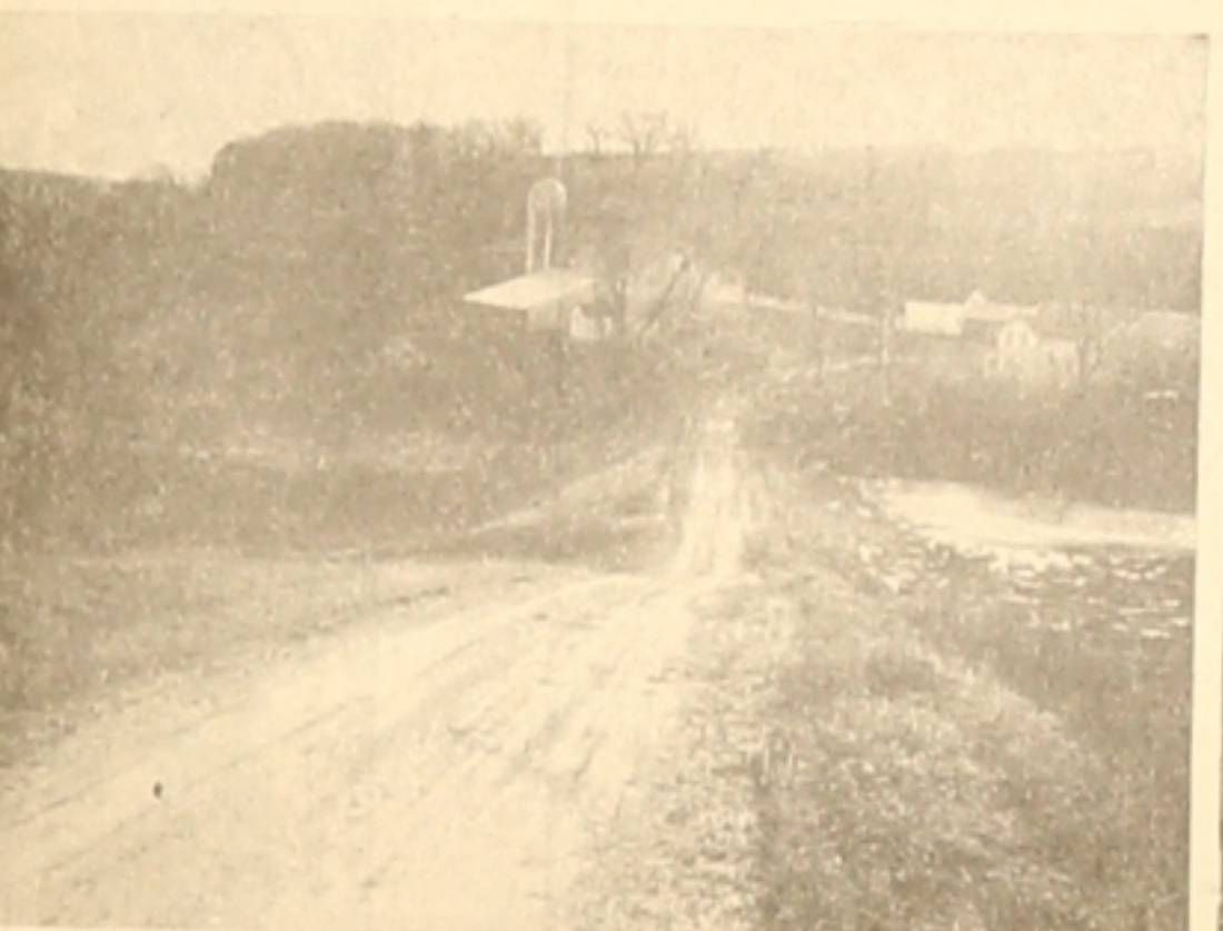
FLORIAN NIENHAUS of Auburn township built this erosion control dam. The dam not only controls a gully but serves as a roadway into the Nienhaus farmstead.
