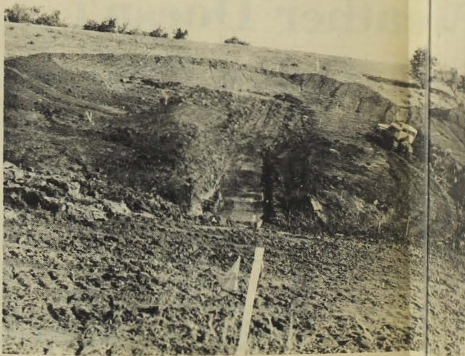
AT WORK: Earth moving equipment is shown at work during the time the one and one-half acre pond was being formed. The
