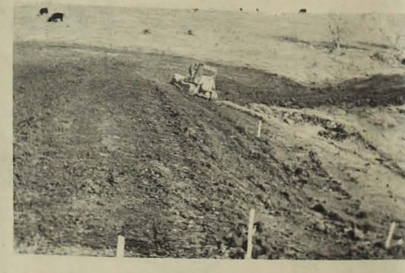
Approximately 10,000 cubic yards of dirt are now in place, making up the dam that will create a 1.5 acre pond. Funds, in the amount
