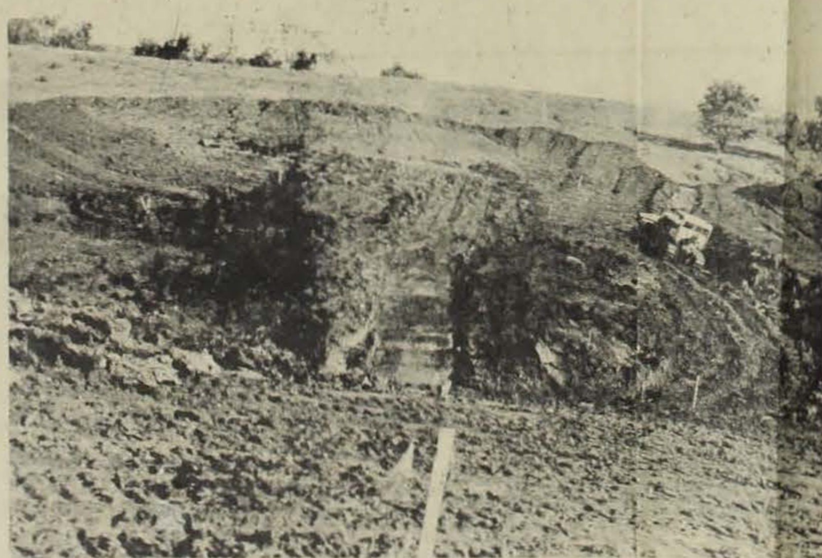
Converting a deep eroding gully at the Clarke Community School into a pond for use by students and teachers as an outdoor classroom, require an extensive construction project. Erik Adams, contractor, is in the early stages building the dam.
