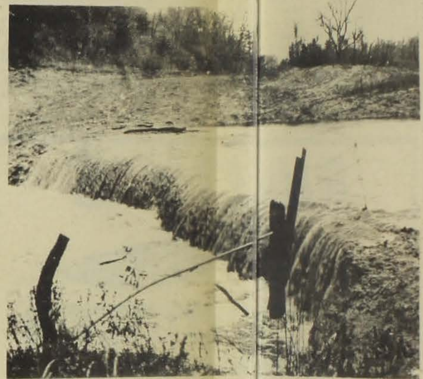
WATERFALL: This waterfall occurred on Joe Ramsey's ground just south of Osceola Thursday morning following a three-inch rain during early morning hours. The water washed away the road bed that was
