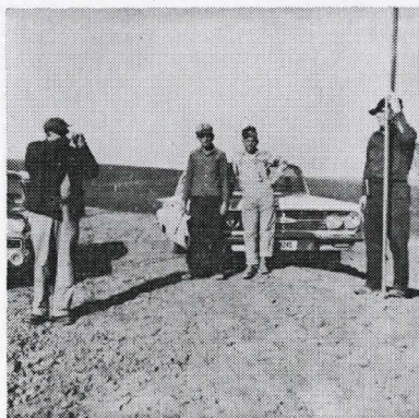
Checking one of the new standard terraces on the Kermit Kincade farm, Cooper Creek Watershed. Left to right: LaVern Whitaker, Cons. Technician, Kermit Kincade, Don Whisler, Contractor, and Joe Luse, State Aid.
