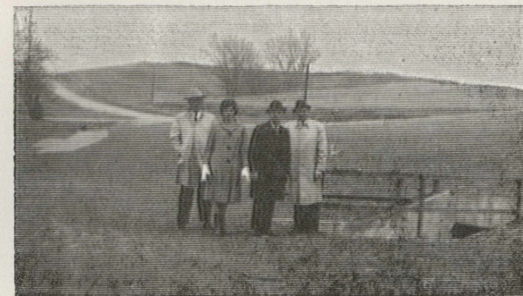
The Pottawattamie County Board of Supervisors making their annual inspection of the watershed structures. They are co-sponsors along with the District Commissioners of the watershed programs in the District.
