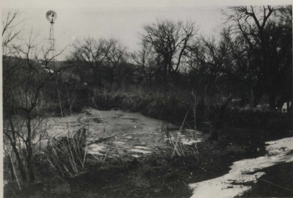
Fill at Sta. 32 + 00 Spillway to Left
