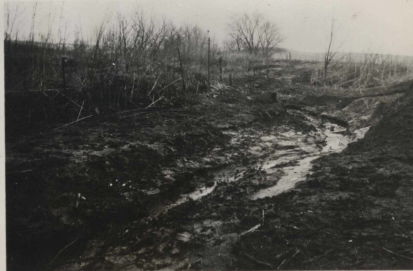
Spillway at Sta. 32 + 00 Looking Upstream
