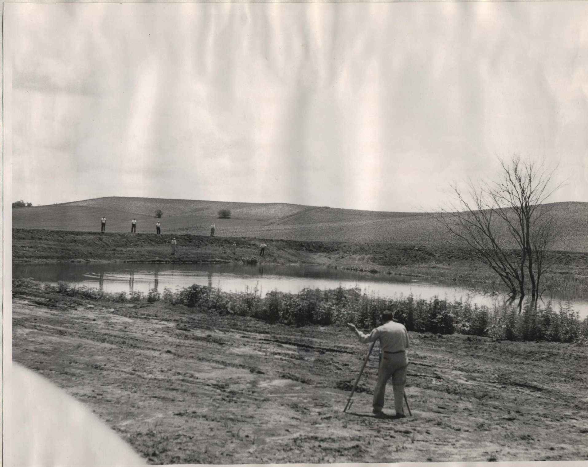
OUR ENGINEERS HELP TO LAY OUT STOCK PONDS. HERE IS ONE OF THE GRONSTAL FARM NEAR TREYNOR
