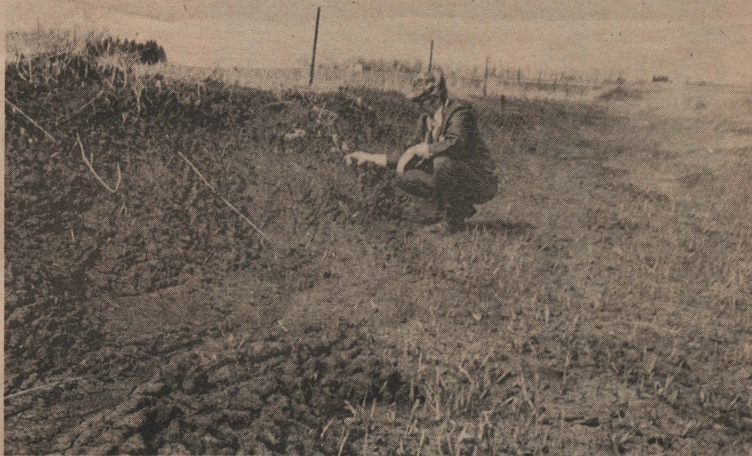
a roadside ditch in dickinson county filled with topsoil blown by the winter winds
