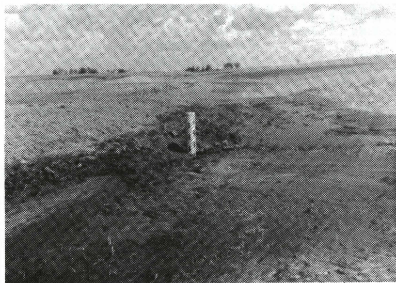
Tile outletted terrace. Lauren Wright farm, 1 mile south-east of Montezuma. The metal culvert pipe drains water into a tile eliminating need of a grass waterway.
