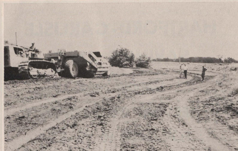
Building Cut and Fill Standard Terrace
