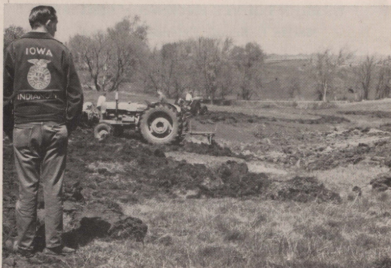
FFA Field Day Shaping a Waterway for Seeding
