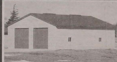
Mark Baumler's new 40x52 storage shed from J&W Lumber.
