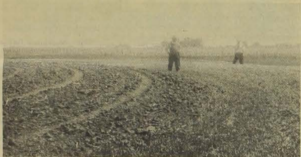
Chester Vigars, chairman of the Hardin County District Commissioners, stands in the channel of one of the terraces he constructed with a tractor and plow in the spring of 1945. Rounds two miles long were plowed in preparing the land for beans above this terrace.
