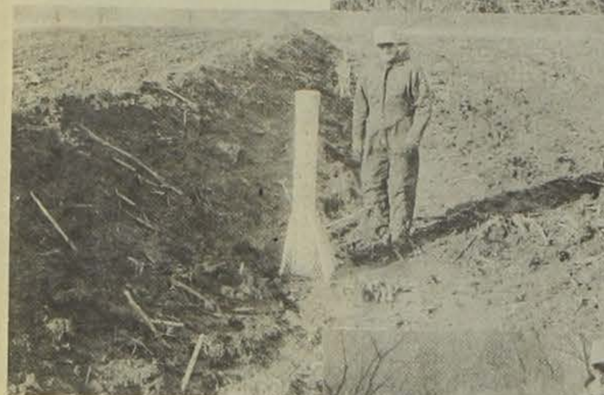
Homer Calkins stands beside a terrace intake which is a part of the terrace system that was installed at Calkins Campus during 1984. Trails are planned so people can walk on the terrace to see how a terrace works. Terraces are a component of a resource management system used on cropland today. SCS designed and laid out these terraces in the same field which SCS laid out a contour line in 1945.
