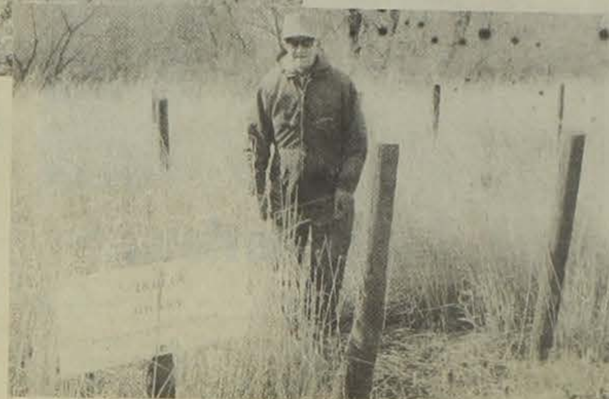
Homer Calkins stands beside a terrace intake which is a part of the terrace system that was installed at Calkins Campus during 1984. Trails are planned so people can walk on the terrace to see how a terrace works. Terraces are a component of a resource management system used on cropland today. SCS designed and laid out these terraces in the same field which SCS laid out a contour line in 1945.
