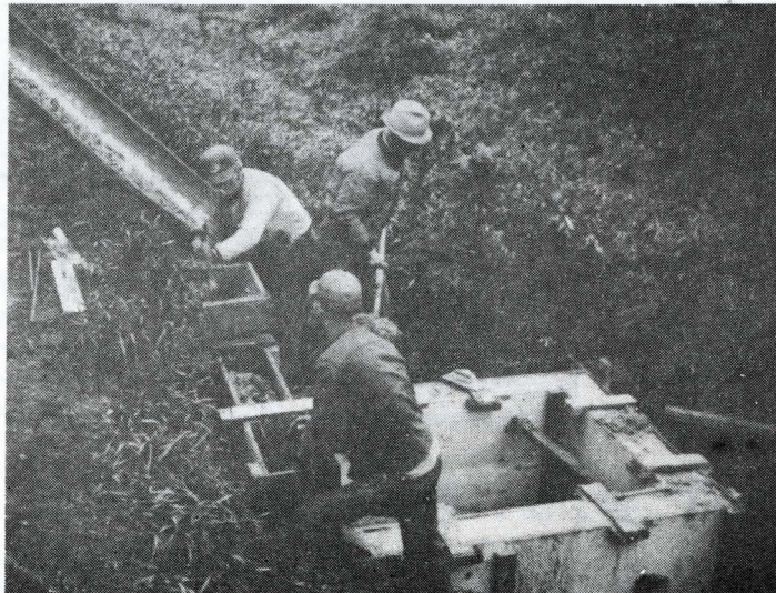
Steve Sholty, is assisted by his father, Art and brother in pouring a reinforced concrete riser attached to a road culvert. The riser will provide gully control upstream in Sholty's farm.
