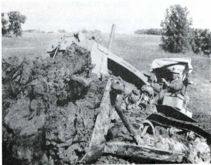
"Pushup" terraces are the style now. Here, Bob Ruser pushes put a terrace on the Murl Sievertson farm north of Ida Grove.
