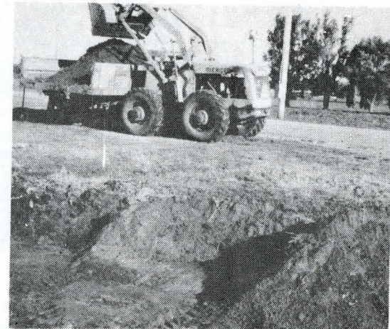
Here, an Ida Grove city maintenance crew man cleans the sediment from a ditch just North of the National Guard Armory.
