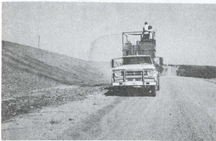
This truck-mounted Hydra-Seeder rented from Cherokee County by Ida County applies a complete seed, fertilizer, and mulch mixture to the steep slopes of the road project southeast of Battle Creek.
