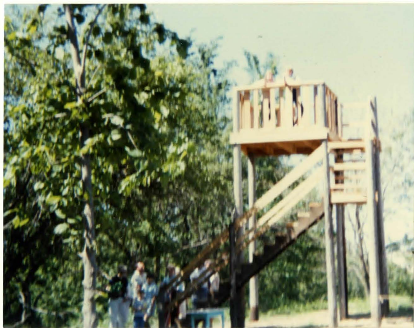
Lookout Tower constructed
