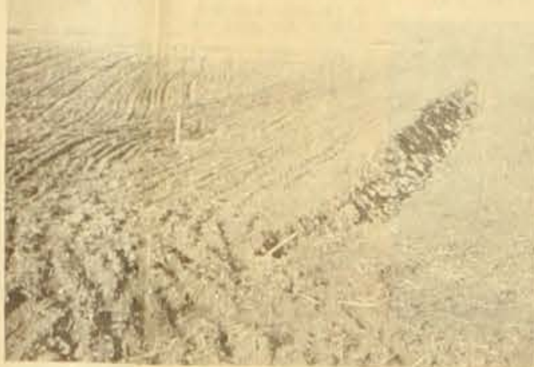
This ground level picture of one of the terraces shows the steep backslope which will be permanently seeded. The intake pipe has holes in it to
