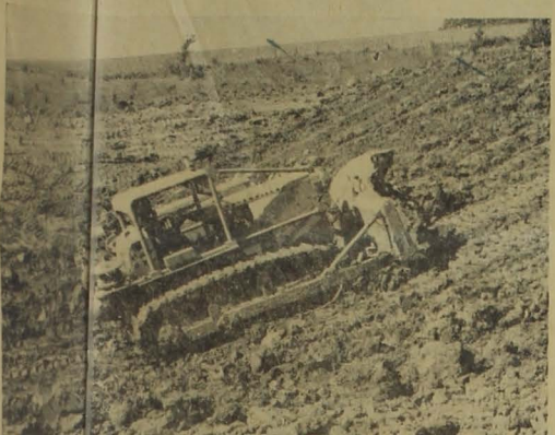
Pond Construction Two catapilla's team up to scoop up earth on a pond construction project on the Floyd Gray farm four miles east of Albia. Pond will be 16 feet deep and requires 2,250 cubic yards of earth to be removed from the fill.
