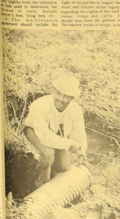
Checking the 10" tile outlet to the Delbert Dan-P. Krieb mutual in Westfield township Technician Bill Baugh of West Union. This system was designed to improve drainage and give an adequate tile outlet for members of the group.
