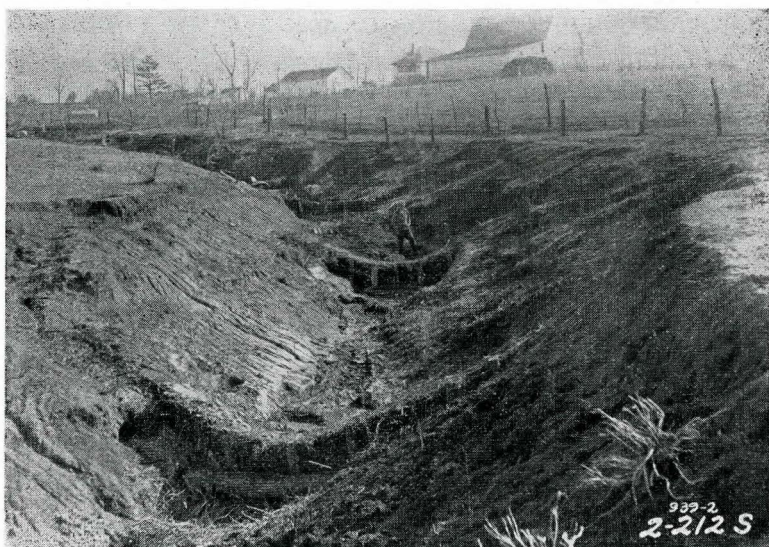
Fig. 6. The gully shown in the picture was threatening the farm of M. P. Christensen of Coin, Iowa, when it was treated by placing wire check dams and willows in the bottom and planting the banks and shoulders to black locusts.
