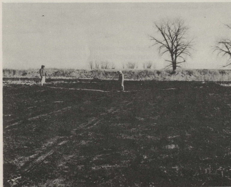
Surface drain constructed on Otto Lorch farm in Westport township. Old tile system was not adequate to carry off excess water. A surface drain was installed. 6 farmers installed surface drains.
