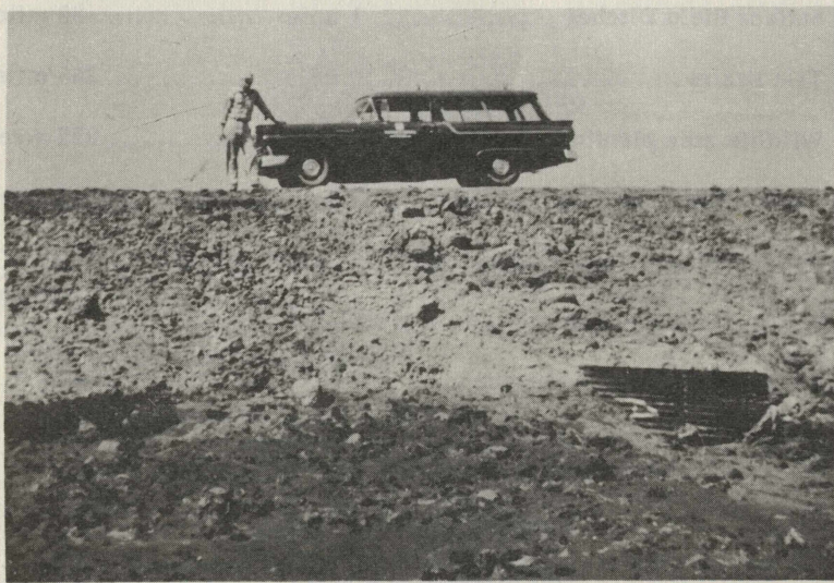
Gully control structure on the Wm. Warnecke farm in Lakeville township. Operated by Larry Bush. Gully had a good start in cutting back into cropland. This is an earth fill structure with a drop inlet.
