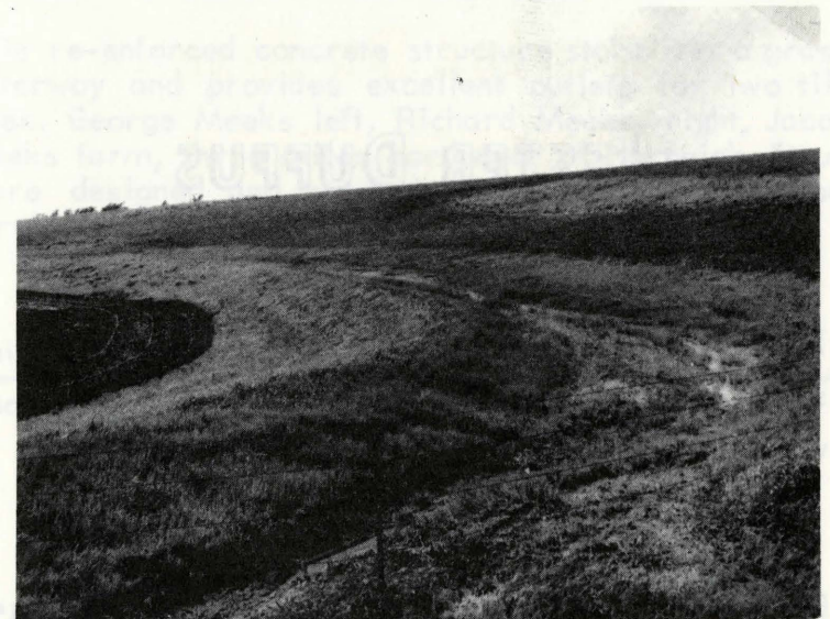
This seeded diversion on the Gertrude Newkirk farm 3 miles north of Malcom, protects bottomland hill overwash. The farm is operated by the McGarry Brothers.
