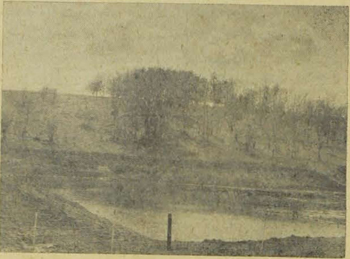
The top picture was taken April 18 on the R. M. Heston farm in Franklin township. Two weeks later the bottom picture was taken of the same area after construction of an erosion control drop inlet dam had been completed.
