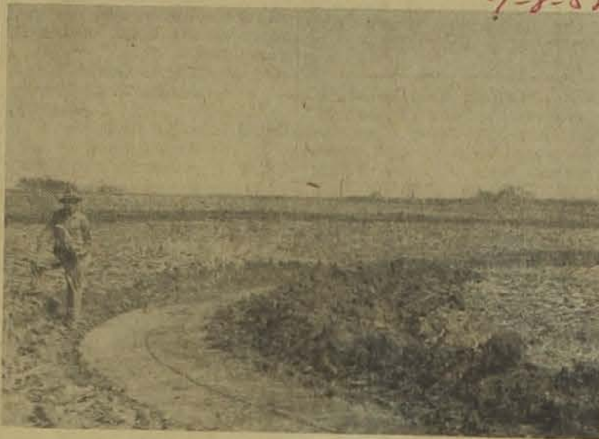
Partially completed standard terraces are shown under construction on a field of the Carl Luce farm in Green Bay township this spring. Harold Anderson, work unit conservationist of the Clarke County Soil Conservation District, demonstrates the terrace depth as it was being built with the use of a road maintainer.
