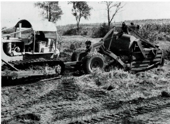
FRANK WOODALL contractor is placing a blanket of reeds canary sod at the end of a newly shaped waterway on the Max Dockendorff farm in Danville Twp. This field, containing sixty acres was also tiled and terraced with tile inlet terraces at this time, tying down another 60 acres of the Geode Lake Watershed.
