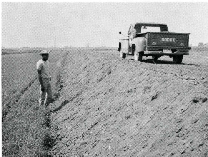
THIS SEEDED BACKSLOPE , tile inlet terrace is located on the property line between the Russell Seymour and Robert Wagner farms in the Geode watershed. Earl Cosby of the SCS is shown checking the design just prior to re-establishing the line fence on the terrace ridge.
