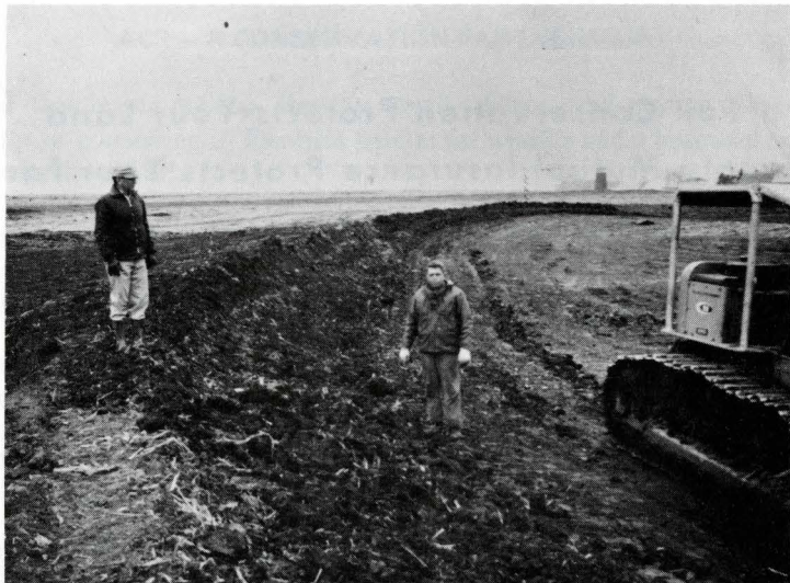
NEARLY 12,000 FEET of parallel, tile inlet terraces were constructed on the Warren Langwith farm in Washington Twp. Harry Bryant, top, SCS and Wendell Wilson, contractor are checking a section of seeded backslope as the terraces are finished up.
