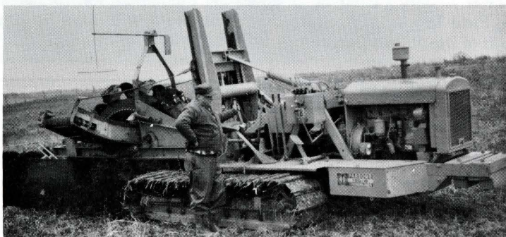
BACKHOE — DRAGLINE — TILING
