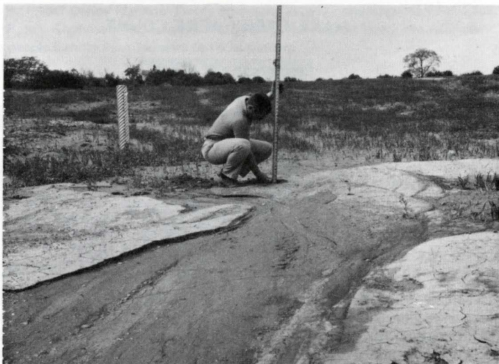
HARRY BRYANT, SCS checks the depth of silt that was desilted from the first heavy rain behind one of Walter Lanes new tile inlet terraces. The top soil would have washed off the farm had the terraces not been there. Years of farming and depositing of silt in the old waterway areas will help level this farm and improve its farmability.
