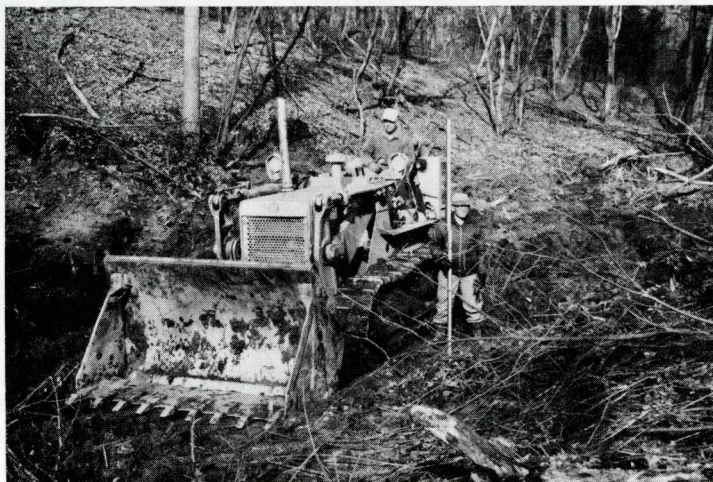
BUCK LA MAR, OPERATOR FOR KINNEY CONSTRUCTION , was clearing the dam site as Harry Bryant, holding the survey rod, helped survey the site for construction of a combination erosion control and wildlife - recreation pond on Carl Schwerin land in Flint River Twp.
