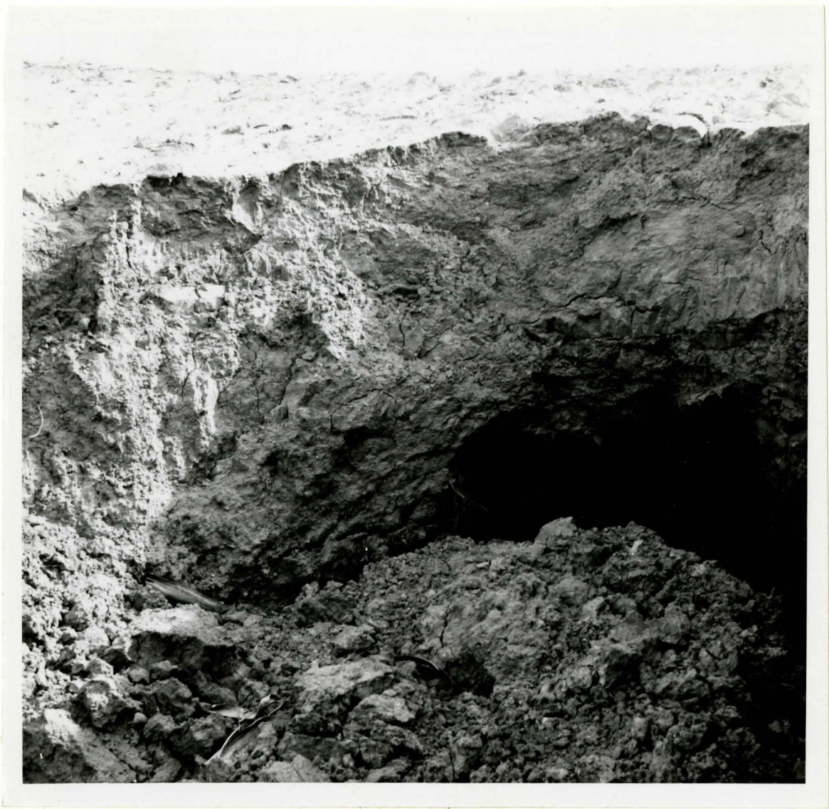
A VOID WHICH PARALLELED THE TUBE, THUS CAUSING THE BLOWOUT.
