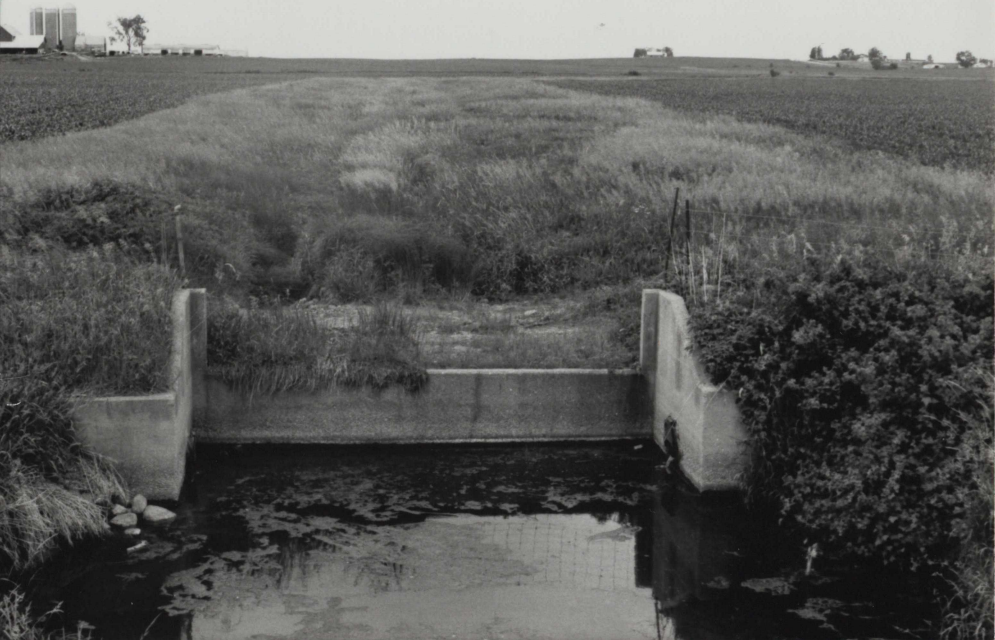
Hoffman/Broghammer concrete structure built Sept. 1959 picture taken 1985
