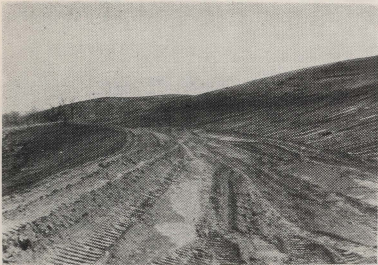
A newly constructed basin terrace on the Bud Ross farm in Hancock Township. The purpose of the basin terrace is to protect the cropland below from the runoff of the steep land above. The area above the basin terrace must remain in permanent grass.
