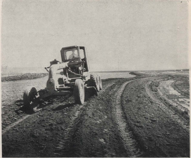
Level terrace being built by a road patrol on the Don Vondrak farm in Garfield Township. This is one of the methods of constructing terraces that is being used in Plymouth District.
