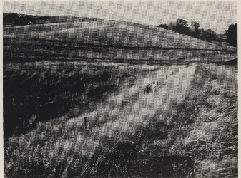
This is the result of establishing brome grass by spreading brome hay on the back slope of this structure. Prior to this the back slope was badly rilled from lack of vegetative cover.
