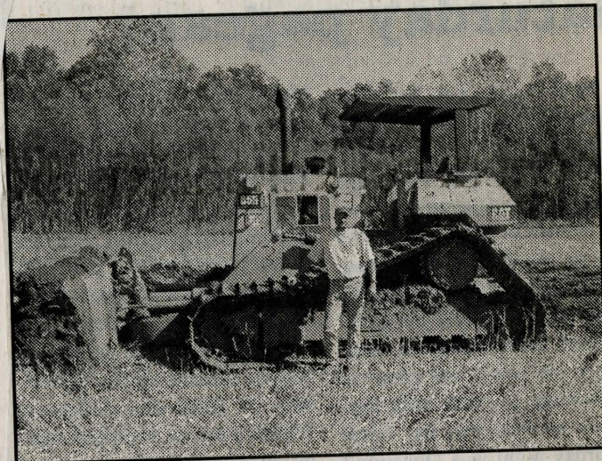
Wapello-Jordie Beeding, owner of River Construction Company, is pictured working on the wetlands restoration projects north of Wapello.
