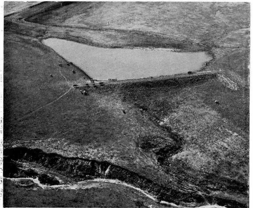
A drop inlet structure, constructed to control erosion on the H. C. and Charles Hansen farm located in Valley township.
