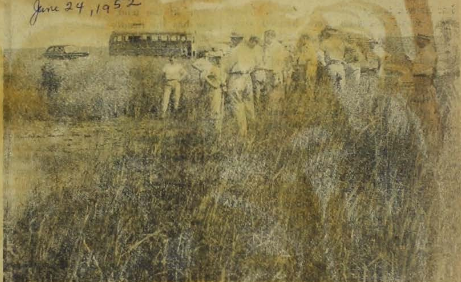
The steps to be taken in the construction of a farm pond were being explained at the D. C. Bollman farm when the above photo was snapped Thursday afternoon. The benefits of farm ponds, both from the standpoint of recreation and water supply, were explained.
