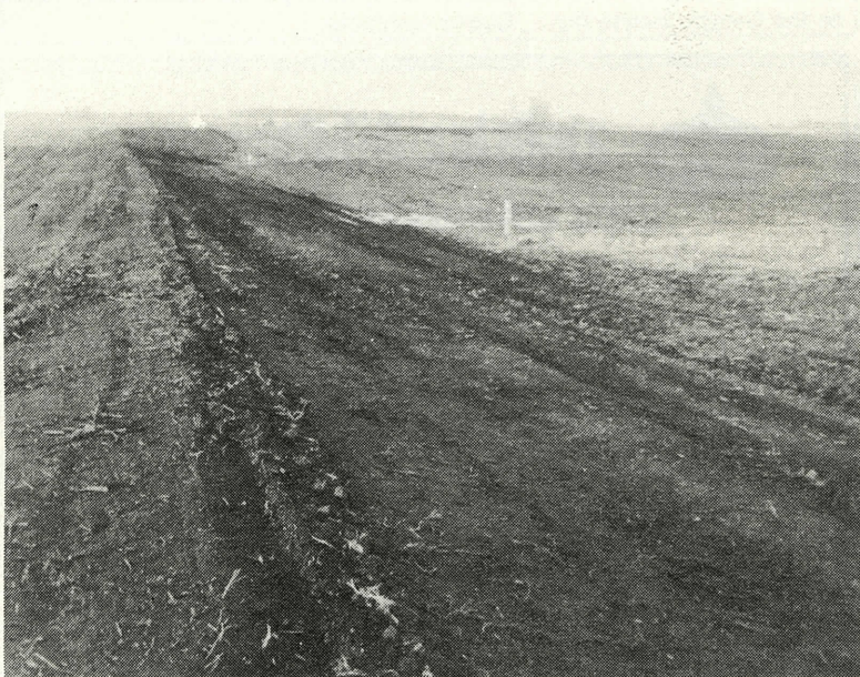
Tile outlet terraces constructed on the George Nopoulos farm. Terraces are the most effective method of controlling water and soil erosion on cropland today.
