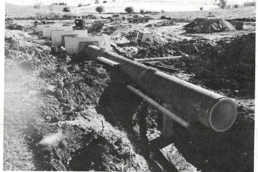
Diamond Lake Watershed structure C-14 shows Bob Owens Construction Company from Newton, Iowa, setting 140 feet of 36" reinforcement concrete pressure pipe diagram which will be used to connect a 3 x 9 drop inlet box to discharge overflow water. Upon completion of structure there will be 24,028 cubic yards of dirt moved which will impound 8 acres of water. Structure is built to keep sediment out of Diamond Lake.
