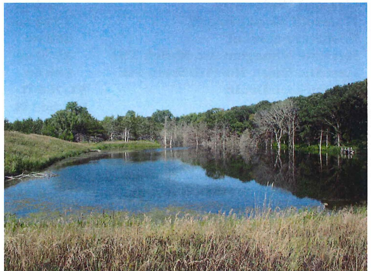
Grade Stabilization Structure funded with Little Sioux Flood Prevention Funds
