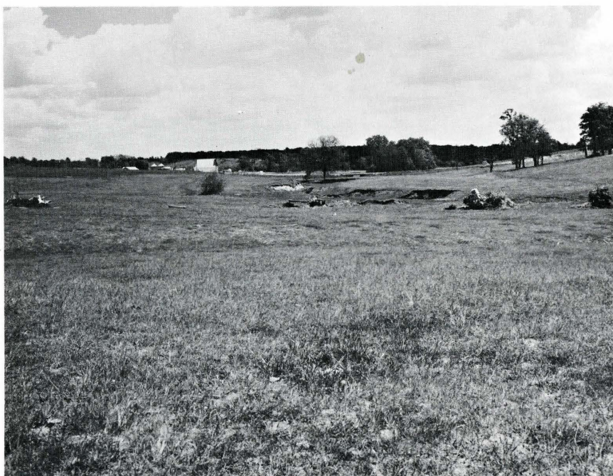
Before Picture — Big Wyacondah Structure Site 8
