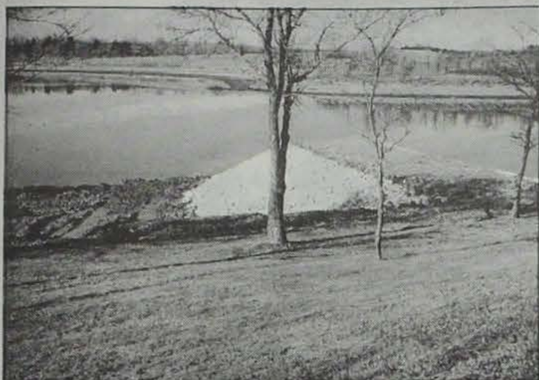
The trees are wired to stakes which can be imbedded in the lake to add stability to the submerged trees, providing fish habitat.
