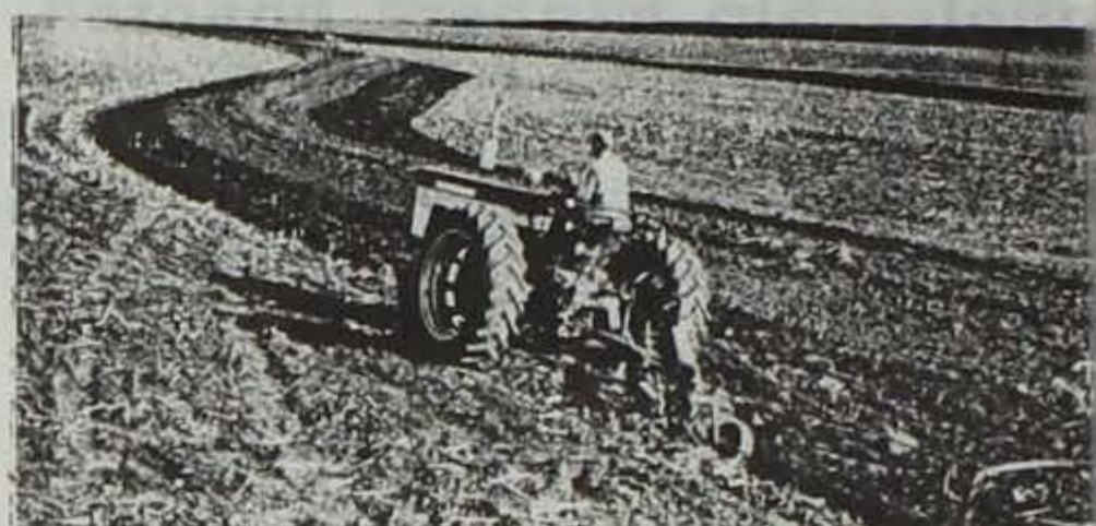
Conventional McCormick one-way moldboard plows do a good job of plowing terrace land. Terraces last indefinitely if you throw the backfurrows on the ridge and deadfurrows in the channel.
