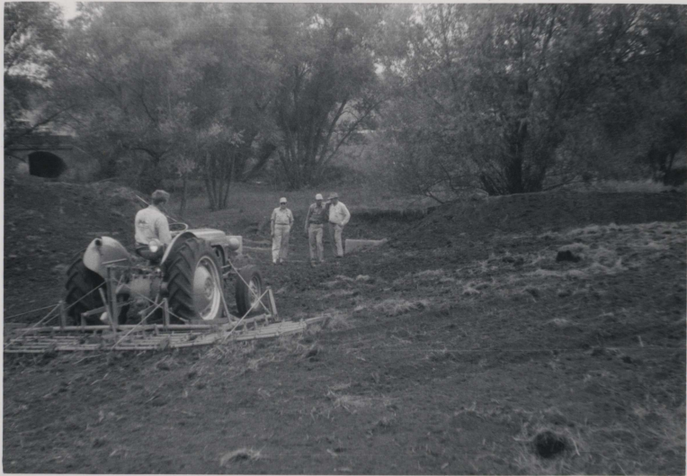
Zearing Field Day - Drop Spillway
