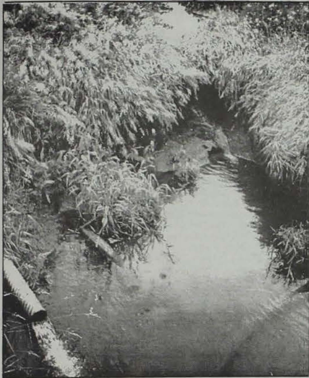
A drop inlet installed at this site in Section 30 of Wright Twp., East Pottawattamie County now controls the damage evident in this picture, taken on the day the area was being surveyed.
