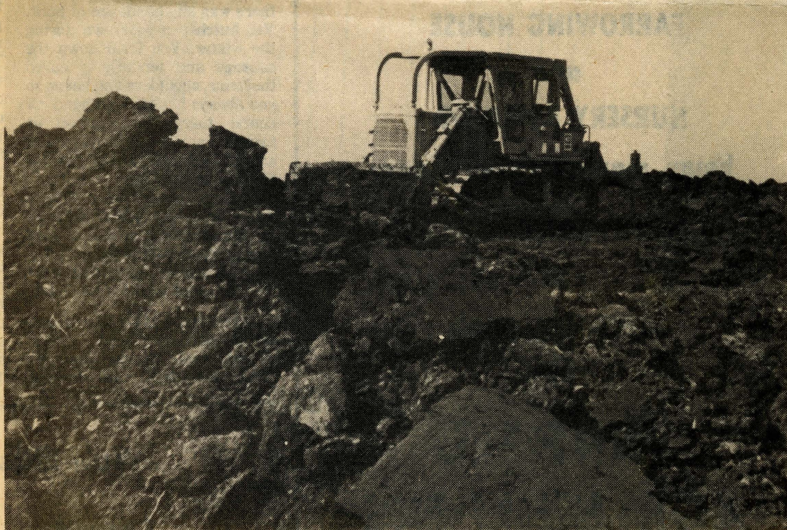
Chuck Allgood's construction crew moves the topsoil from a stretch of land on the Eric Massner farm in preparation for constructing another terrace. The topsoil will be moved back to its original position after the fill has been added for the proper sloping of the terrace.
