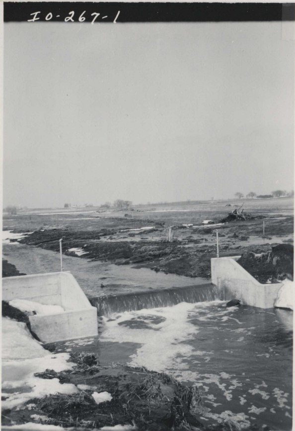
Hoffman/Broghammer concrete structure built Sept. 1959 picture taken 3/31/60
