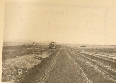
TERRACES —Round hay terraces with farmstead backsheds were constructed on the Carl and Laker Becker farm in Putnam township. Water held by the terraces is drained through surface in-take into the lines.
