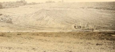
EROSION CONTROL —An erosion control dam was built to control a gully and protect a driveway on the Richard Jensen farm in Pleasant Valley township. The dam is shown during construction.
