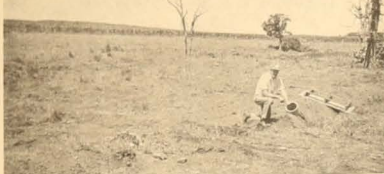
TILE—Low Redensetter and four neighbors in Ashura township cooperated to install metal tile drains. Outlets to drain wetland from a 250 acre watershed will be provided by the main tile.
