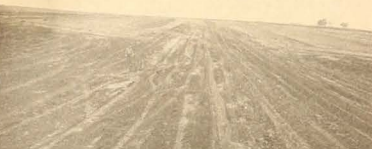
COMPLETED —Completed terraces on the Becker farm are straight east-west. Average slope of the field is only 3-4 per cent but slopes were exceptionally long. The terraces will reduce slope length and thereby prevent topsoil, fertilizer, and chemicals from leaving the field.
