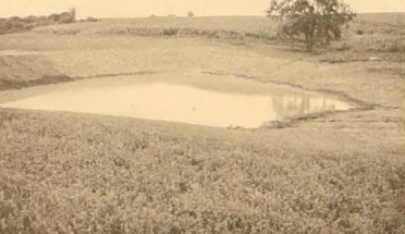
WATER POOL —The permanent water pool on the Jensen dam is beginning to fill soon after completion. Terraces on fields in the watershed will protect the structure from excessive sedimentation.
