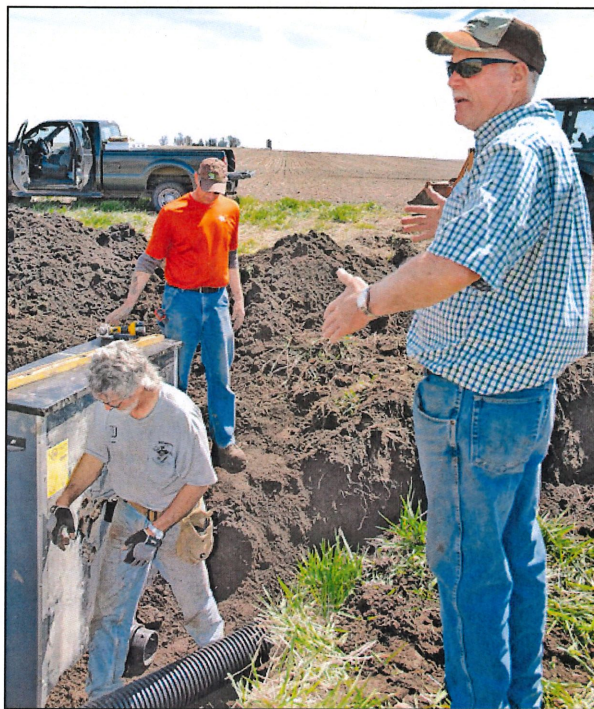
Nick Meier supervises installation of a bioreactor on his farm last summer. The bioreactor will filter drainage tile water from about 40 acres of land in the Miller Creek Watershed. FILE PHOTO
