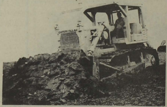
Larry Wallace, employee for Meier Construction of Battle Creek, operates a D-7F Cat bulldozer while building a terrace.
