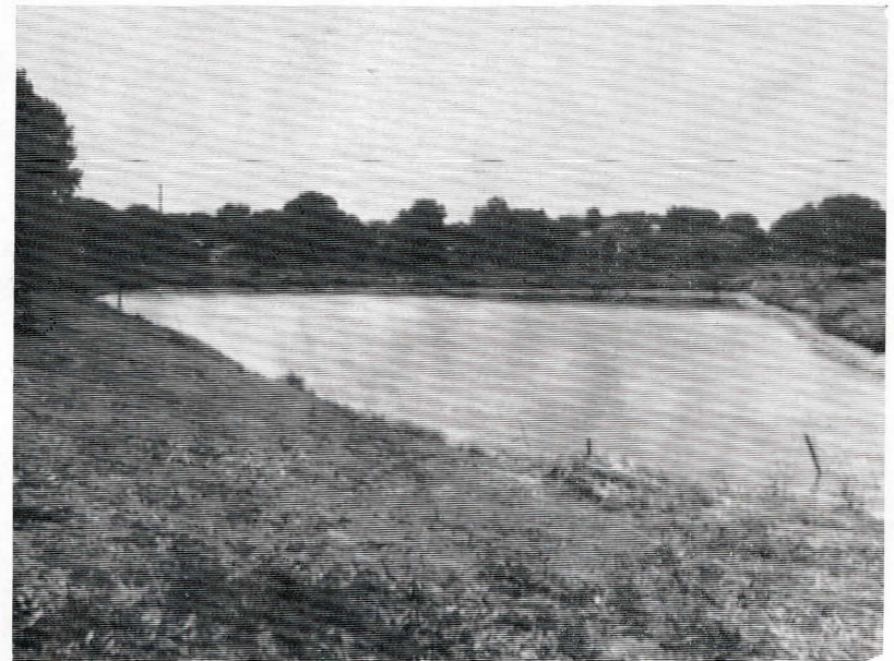
An erosion control pond on the Everett Anderson farm and within fifty feet of the house. The pond controls an overfall at upper end and is outletted thru metal pipe.
