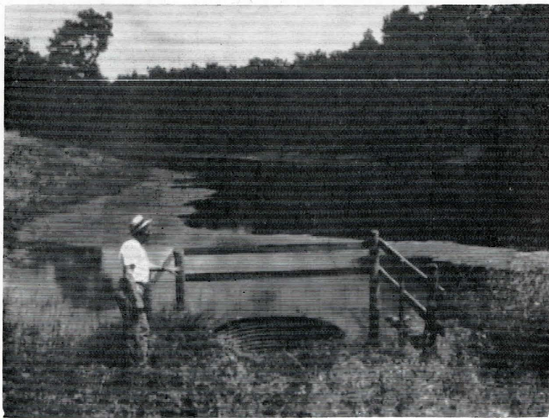
Pond of water almost \frac{1}{4} mile long made by putting a riser on a road culvert on the Harry Lucas farm. The tube is seven foot in diameter.
